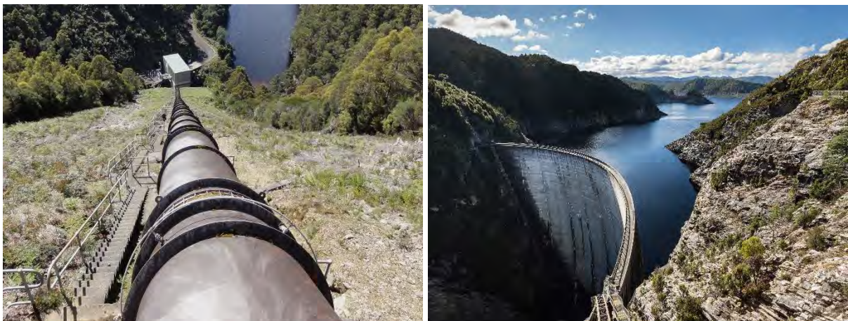
Two hydro-electric plants in Tasmania. Left. Wilmot power station, 32 MW. Water flows down the pipe to the turbine in the building at the bottom. Right: The Gordon Dam, 450 MW. Three underground turbines are fed from an 80 m vertical channel from the bottom of the lake. Credit: Hydro Tasmania
