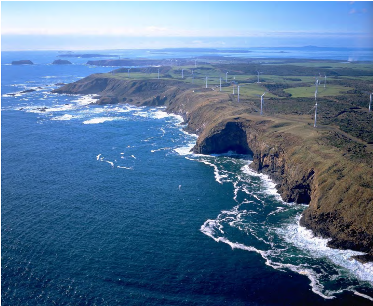
The 140 MW Woolnorth Wind Farm on the far north-west coast of Tasmania. Credit: Hydro Tasmania
